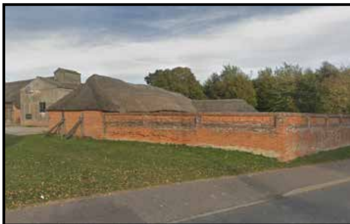
Traditional brick boundary wall
