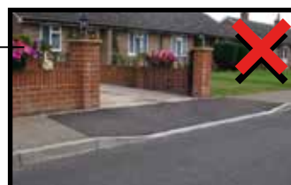
Interrupted pavements over driveways
